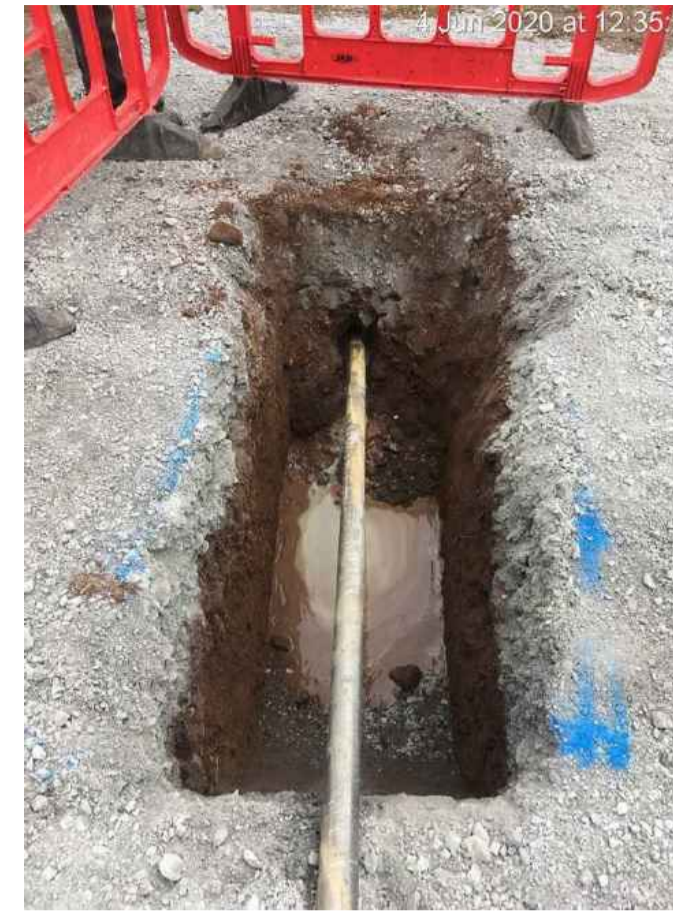
Image 2 : Standard Launch and Receiving Pits
