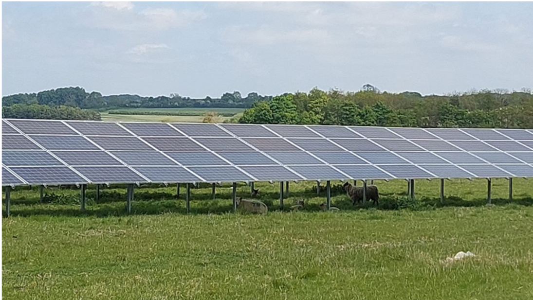
Plate 1: Typical Solar Panel Arrangement – Landscape Formation
