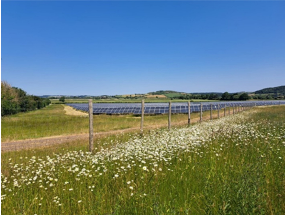
Plate 4: Typical Post and Wire Security Fencing
