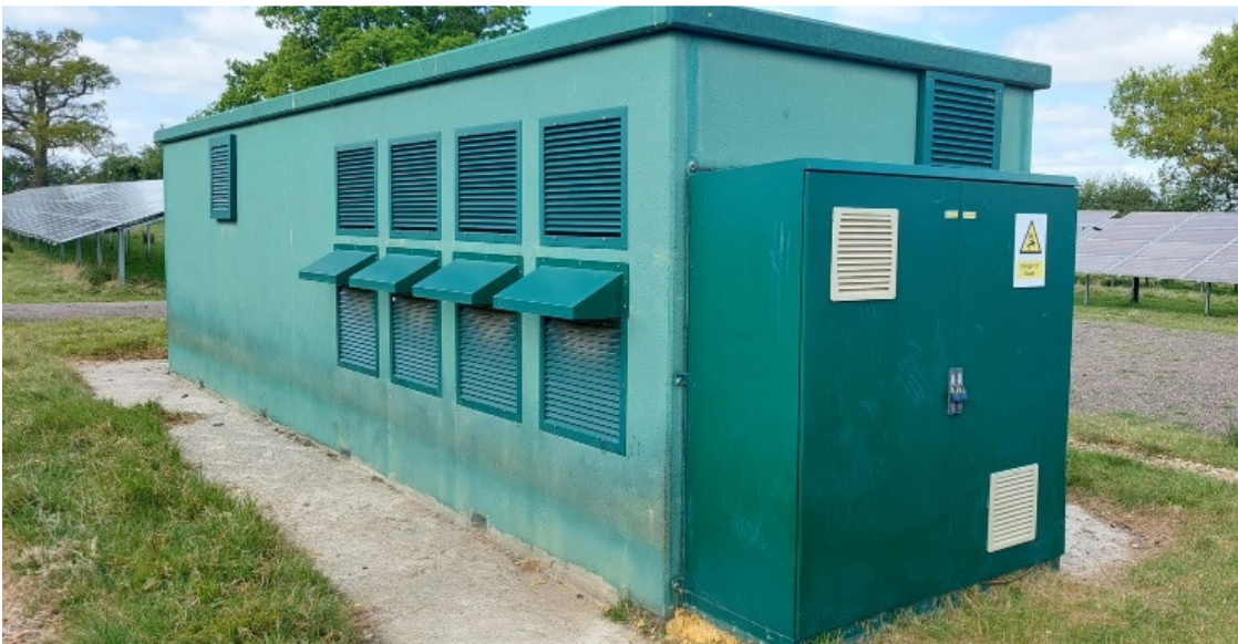
Plate 3: Typical Inverter Container Unit
