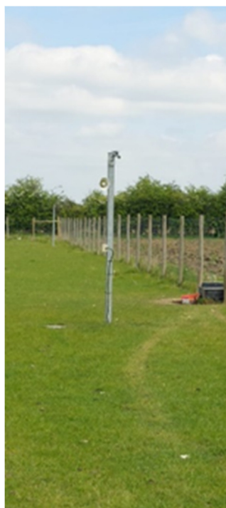
Plate 5: Typical CCTV Camera
