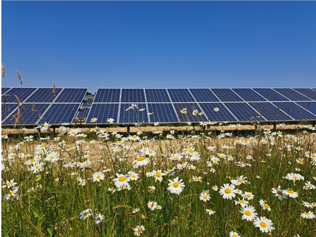
Plate 2: Typical Solar Panel Arrangement – Portrait Formation
