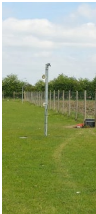
Plate 4: Typical CCTV Camera
